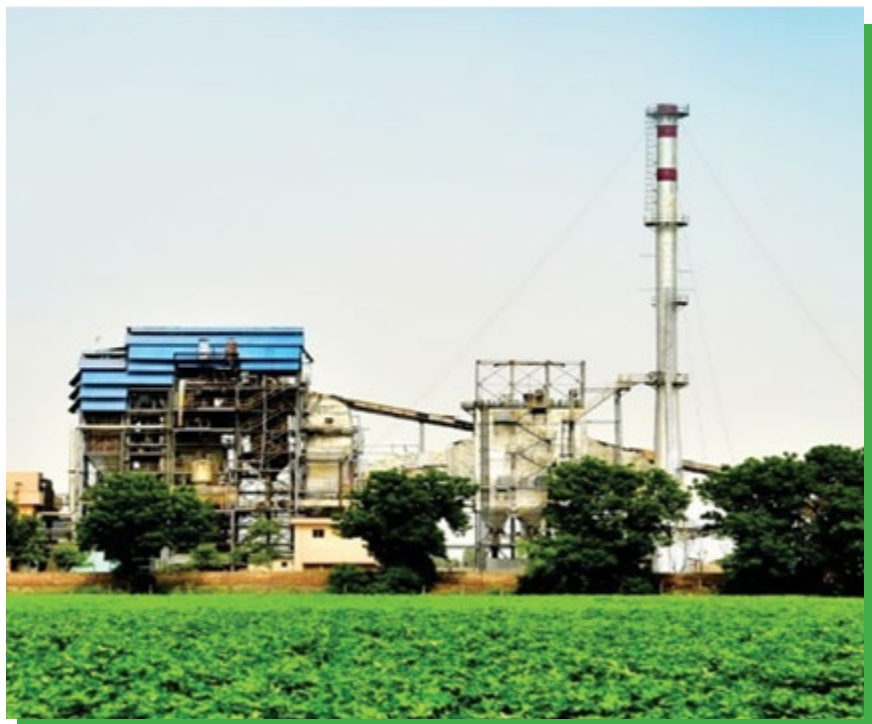
Biomass based power generation plant at Padampur (Rajasthan)
