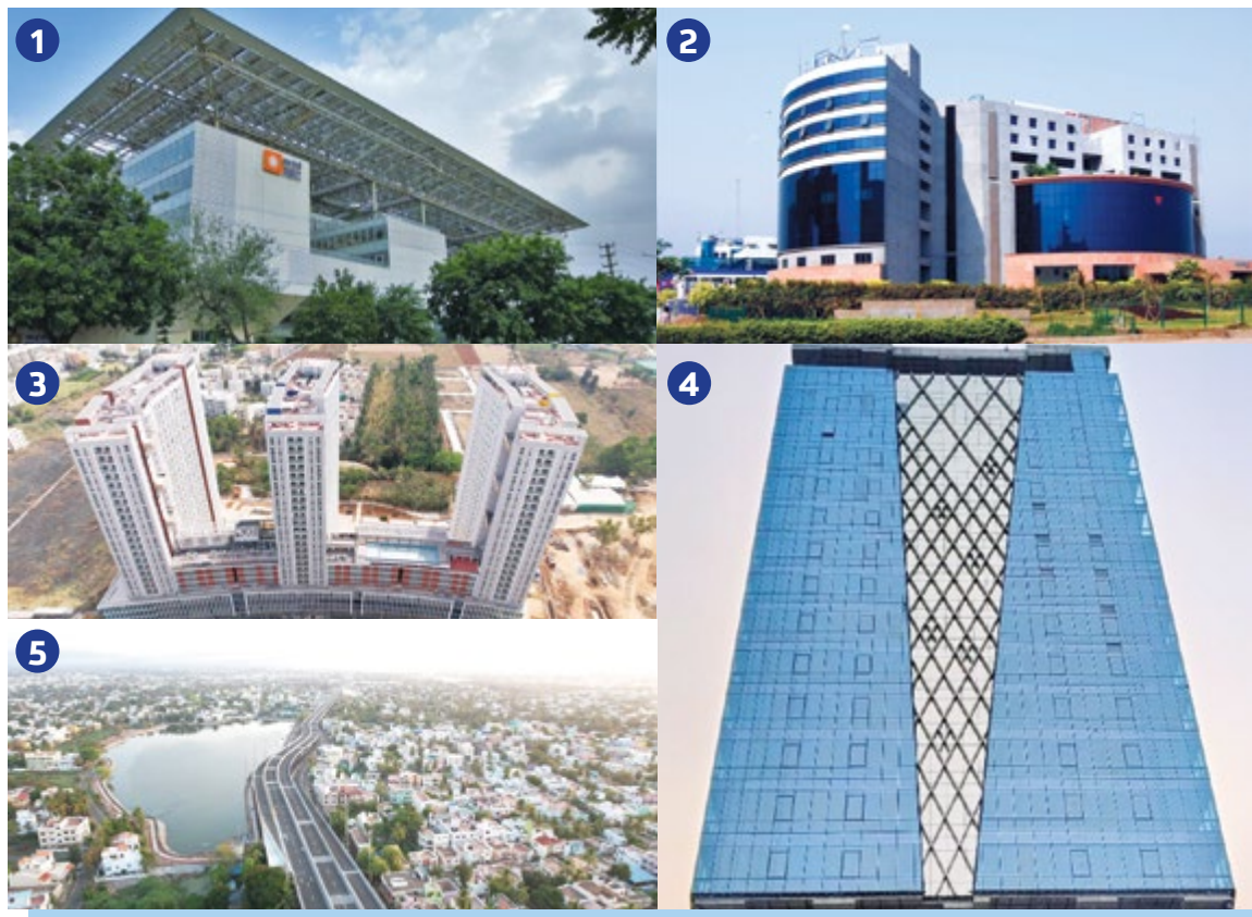
1 Rural Electrification Corporation World Headquarter | 2 Asian Heart Institute, Mumbai | 3 BCUP, Bengaluru | 4 HDFC bank, Kolkata | 5 Vellore Institute of Technology
