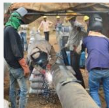
Thumbli Water Pipeline– Cairn Energy India – Rajasthan
