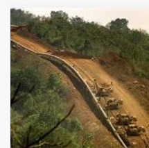
Panvel Dabhol Pipeline Project–Gail Ltd - Maharashtra
