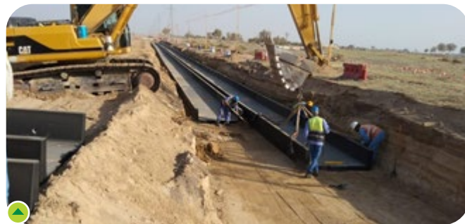
Underground cabling works in Dubai
