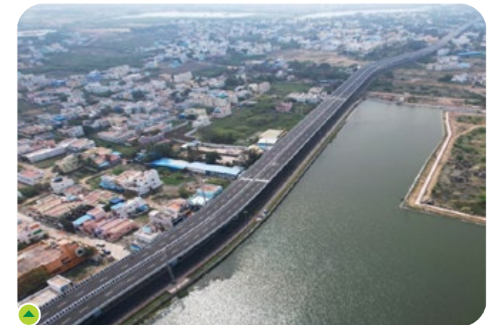
Madurai Chettikulam Flyover, Madurai
