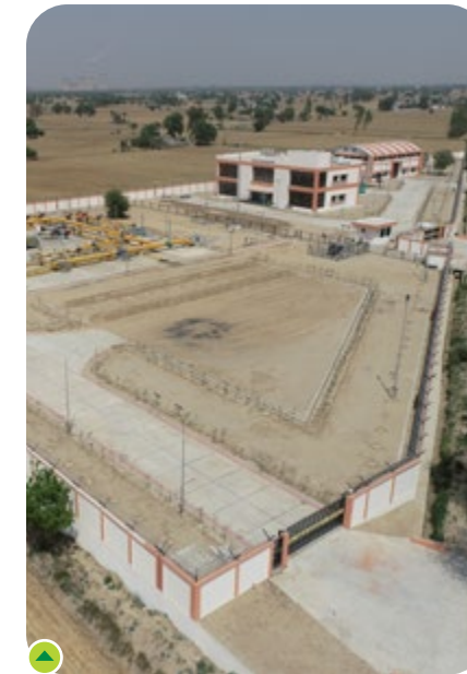
Mallavaram-Bhopal-Bhilwara-Vijaipur RFCL Connectivity Pipeline Project
