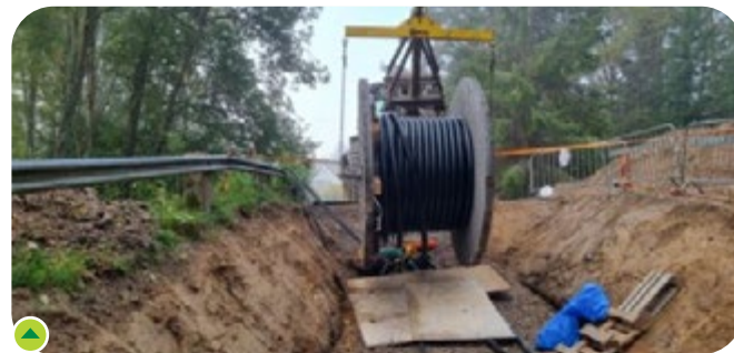
Underground cabling works in Sweden
