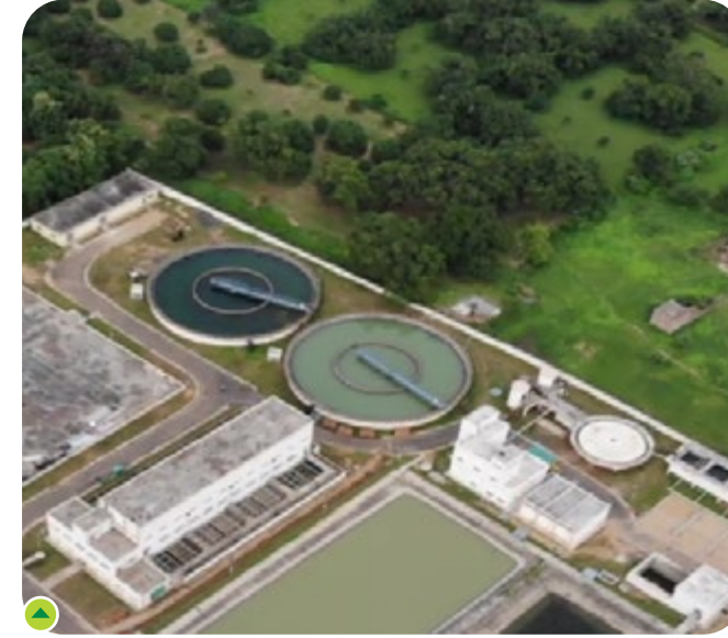
Multi villages 30-50 MLD Capacity Surface Water Supply Scheme (792 km), Bihar
