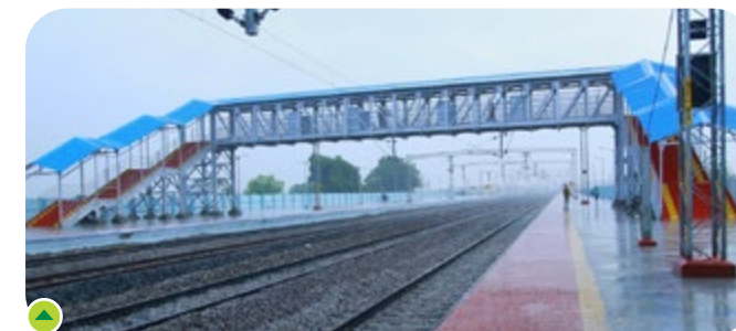
Umdanagar Mahabubnagar Doubling Project
