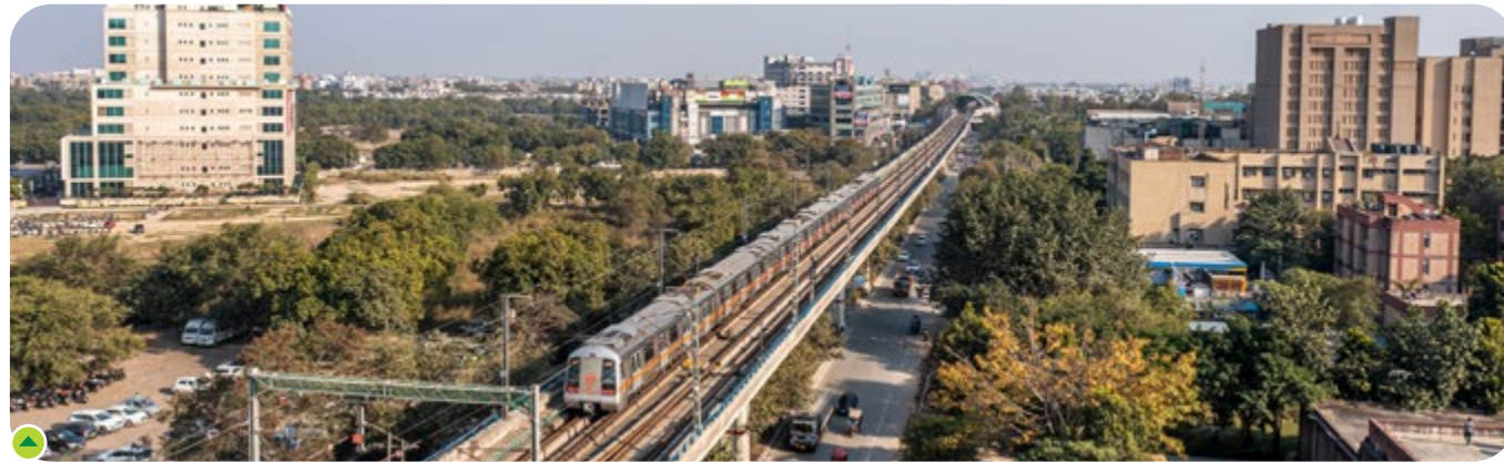
Bhopal Metro project
