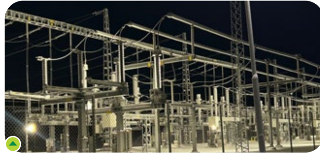
Substation Works in Sweden
