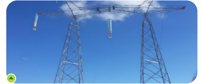
750 kV S-C 353 km Transmission Line in Ukraine
