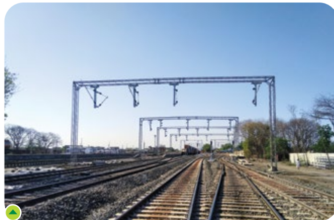
Palanpur-Samakhiali railway electrification project
