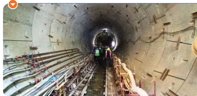
Underground Metros, Bhopal & Kanpur
