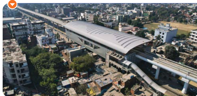
Elevated Metro, Kanpur
