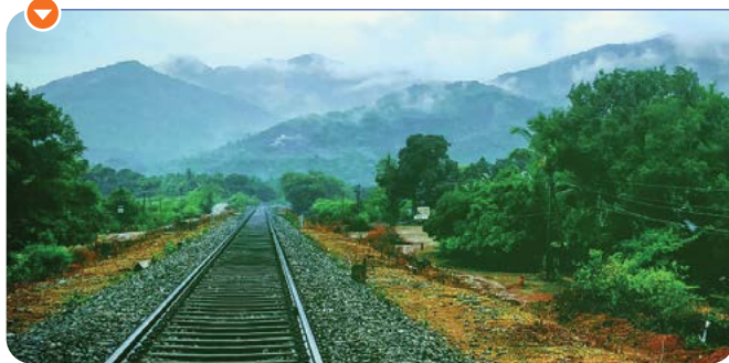
Verna Thokur Railway Project: Konkan region
