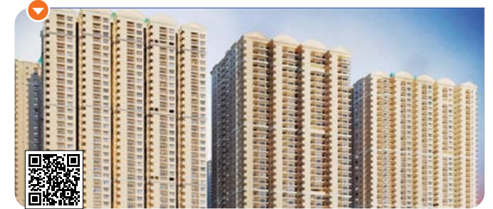
Prestige City - 14 Million square feet of residential building project on design built basis, at Hyderabad
